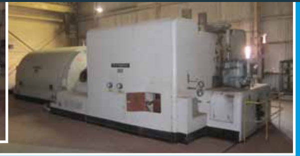
(2) Steam Turbine Generators
