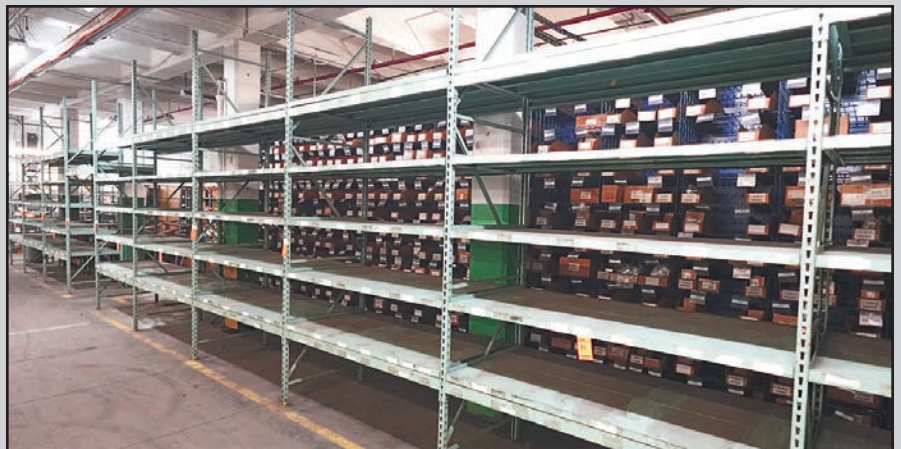
SAMPLE PALLET RACKING
