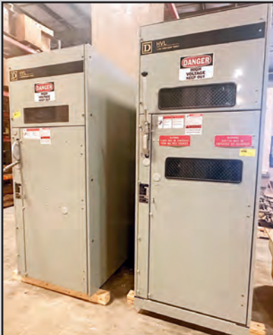
SQUARE D HVL LOAD INTERRUPTER SWITCHES
