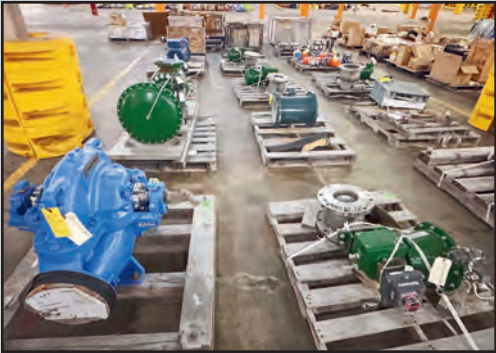
PALLETS OF ASSORTED VALVES, FLOW CONTROLS, MOTORS, PUMPS
