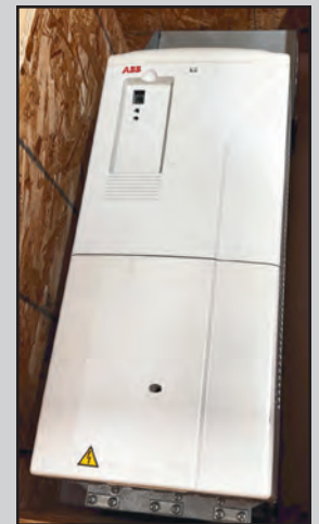
ABB DC DRIVE CONTROL
