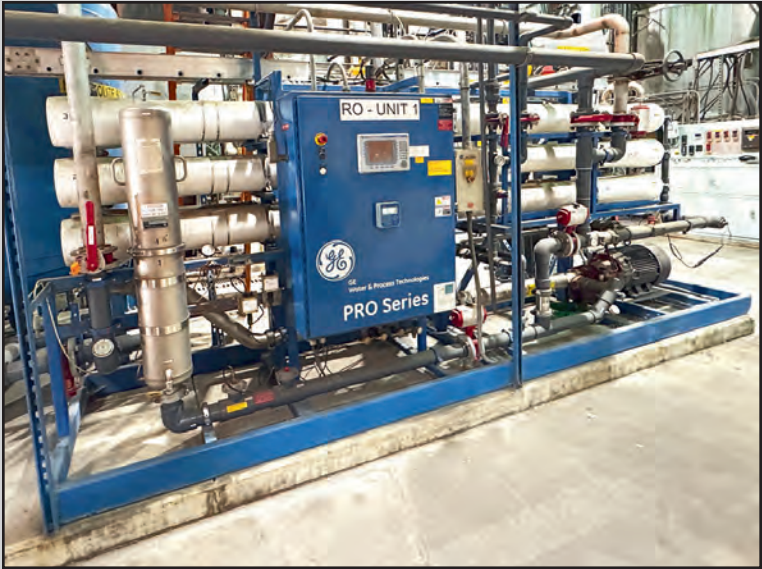
(1 OF 2) GE PRO SERIES 100 GPM RO SYSTEMS
